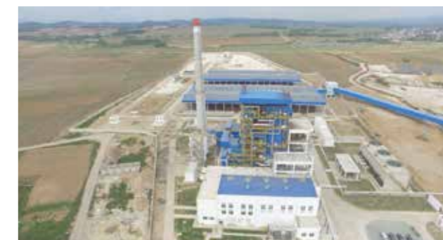
Boiler of Shanghai Electric
