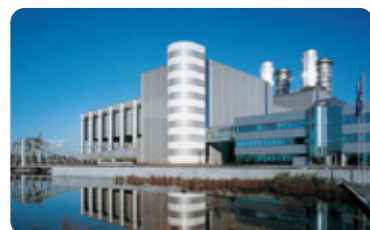
Bruges Power Plant with A-frame ACC in Belgium
