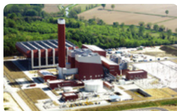
Italian Combined Cycle Power Plant ACC
