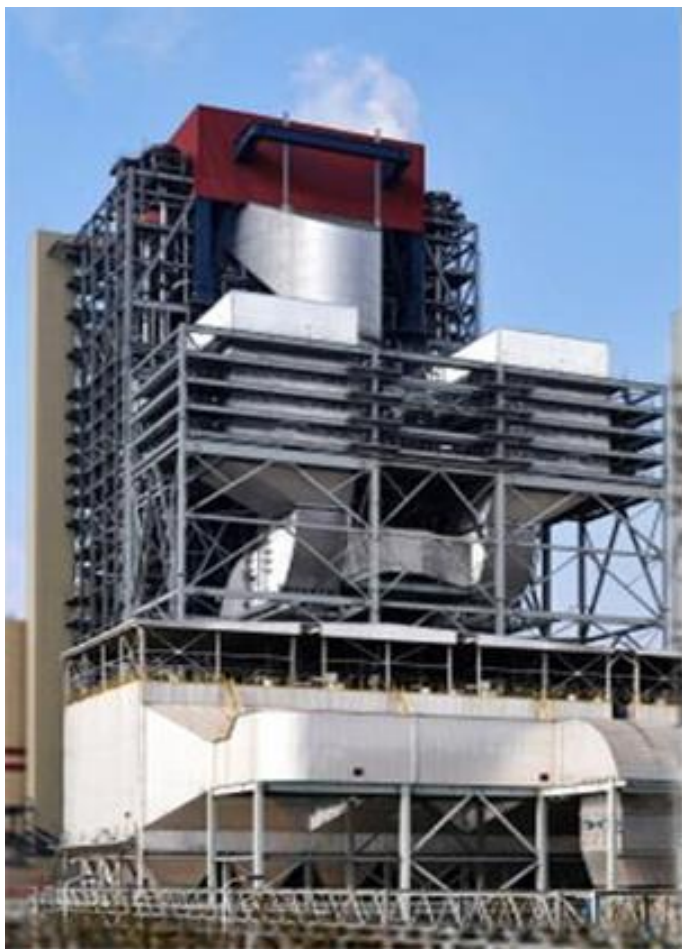
Waigaoqiao 2 Power Plant 2X900MW Retrofitting Project
