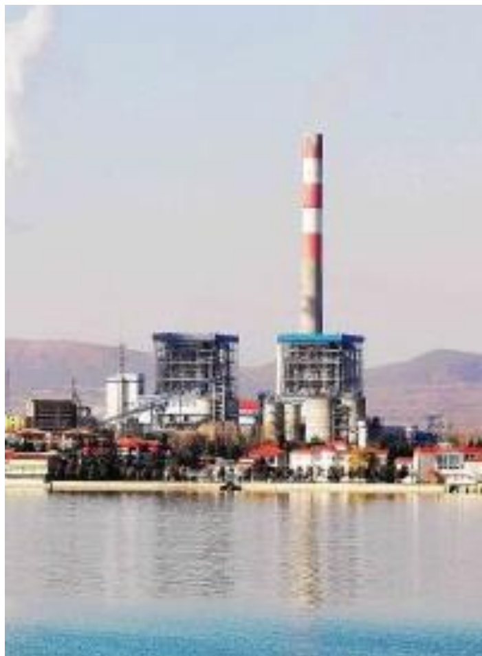
Yaomeng Power Plant 2X600MW Retrofitting Project, High Ash Time of Commission: Jan, 2013
