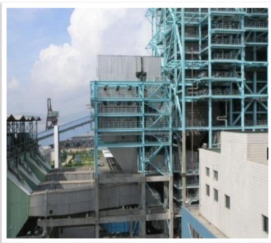
Songyu Power Plant 2X300MW Retrofitting project, First Domestic SCR
