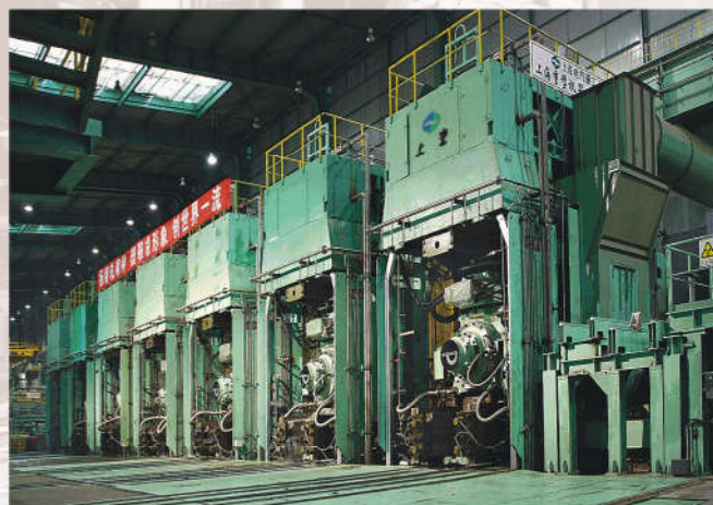
精轧区 Finishing mill section
